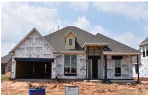
Single-Family Residential Under Construction
