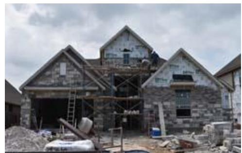
Single-Family Residential Under Construction
