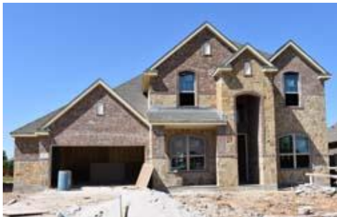
Single-Family Residential Under Construction
